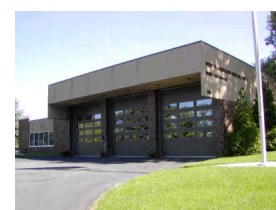
Station B Susquehanna and Twining Roads Dresher PA 19025
